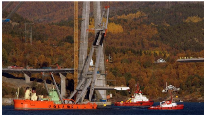
Construction work and inshore assistance
