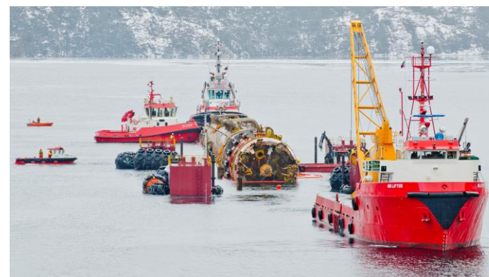
Decommissioning of offshore structures
