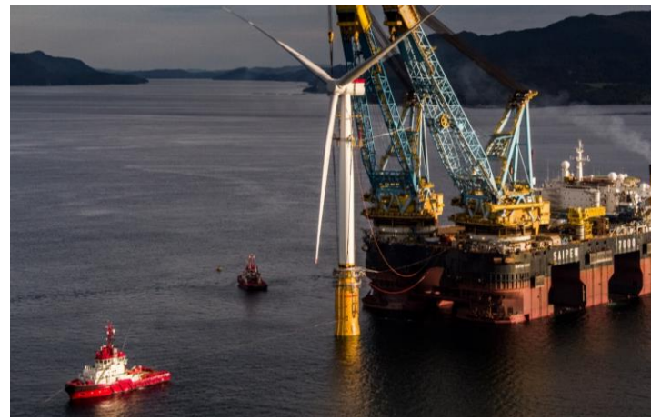
Assembly and installation of wind power
